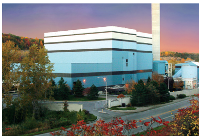
Covanta Onondaga energy-from-waste facility.
